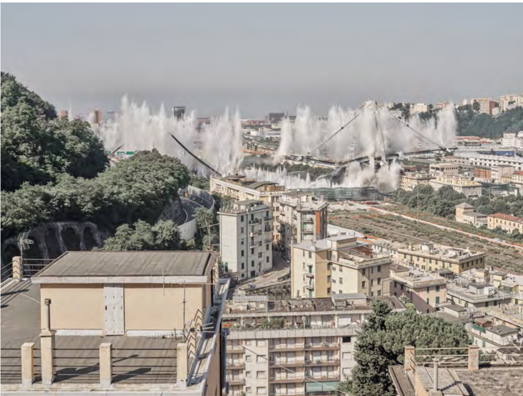
Source: Marco Menghi, Morandi Bridge (Genoa), demolition, 28-06-2019. ©Marco Menghi
