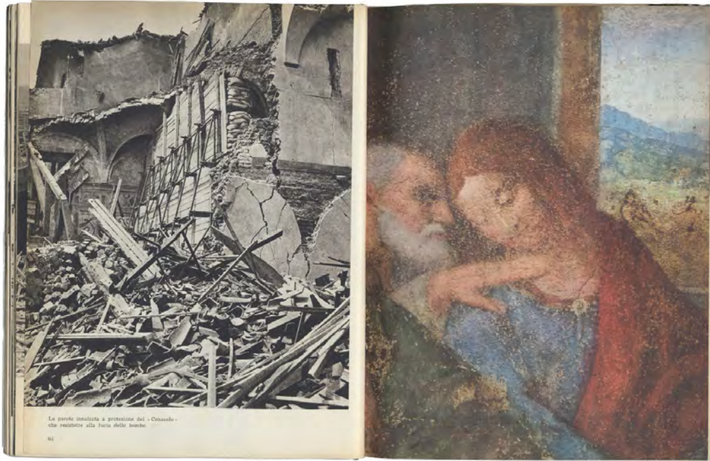
Source: The protective wall of Leonardo Da Vinci's Last Supper erected during the bombing of World War II. In Ronza, Robi. 2002. Milan 1940-1955. Bombed and rebuilt. Milan: Comune di Milano, 64-65.
